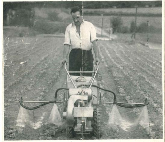
High Pressure Spraying Equipment for rowcrop, bush or orchard spraying.
